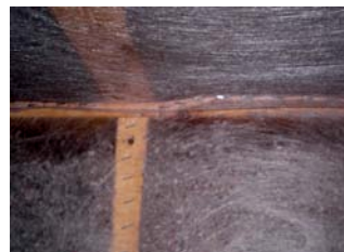
Settling in loose fill wall insulation when installed behind air and moisture permeable netting.
